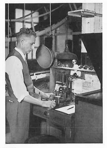
Early in its career, the MAZDA lamp is subjected to rigorous tests and inspections. Even the empty bulb must sometimes pass as many as 15 tests before it is qualified to wear the G-E monogram. Here bulbs are shown at Pitney Glass Works, in Cleveland, undergoing rigid preliminaries, necessary to prove they are "in good shape" to progress to one of our lamp factories and in due course, pass the rest of the 480 tests required of a finished MAZDA lamp.
